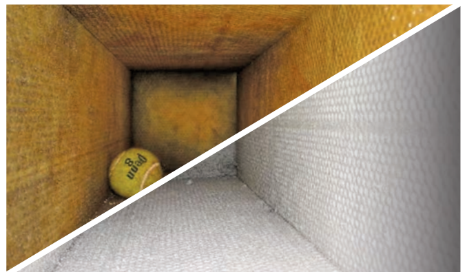
Fiberglass Duct After PURE-Duct
