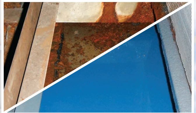
Drain Pan After PURE-Liner 2.0
