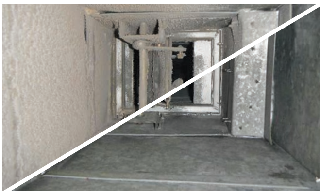
Outside Air Damper After PURE-Duct
