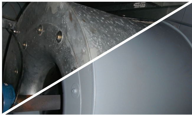
Blower Wheel Housing After PURE-Coat
